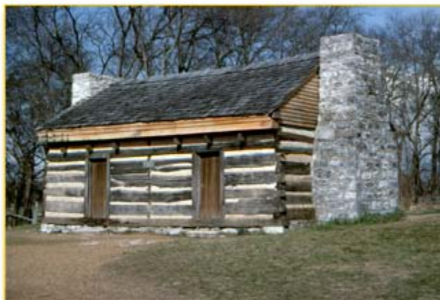
This double-pen log house has fieldstone exterior chimneys at both ends.
