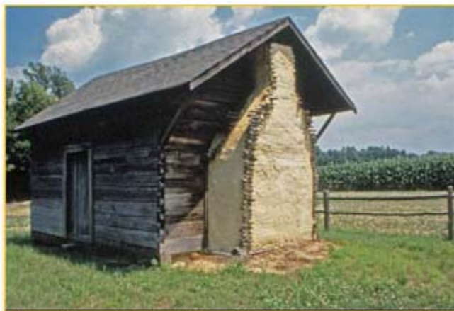
The wattle-and-daub chimney of this single-pen log cabin is located under the eaves for protection from the elements.
