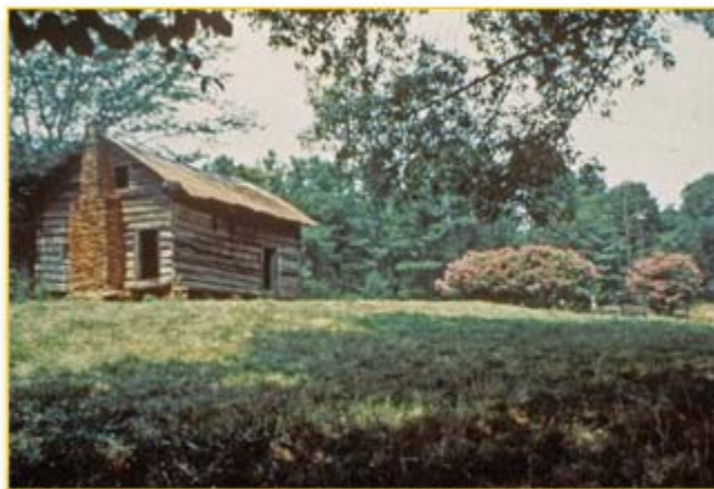
This single-pen log cabin is a Scots-Irish prototype. The small upstairs windows provided light for the sleeping loft.
